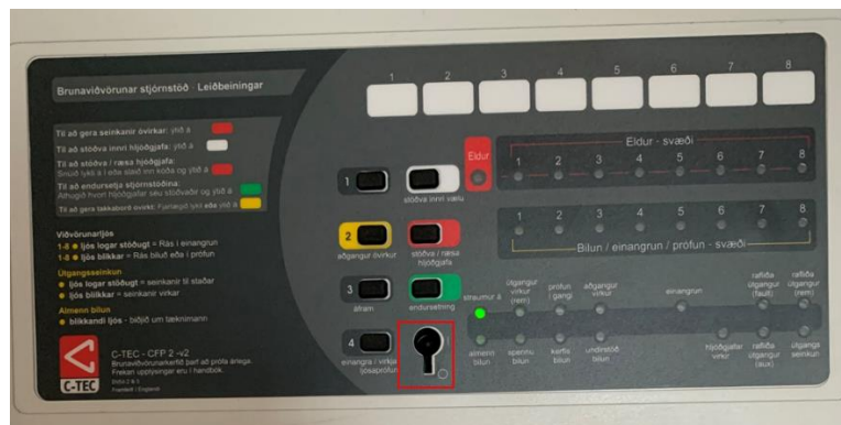
Figure 12 Fire alarm panel.
