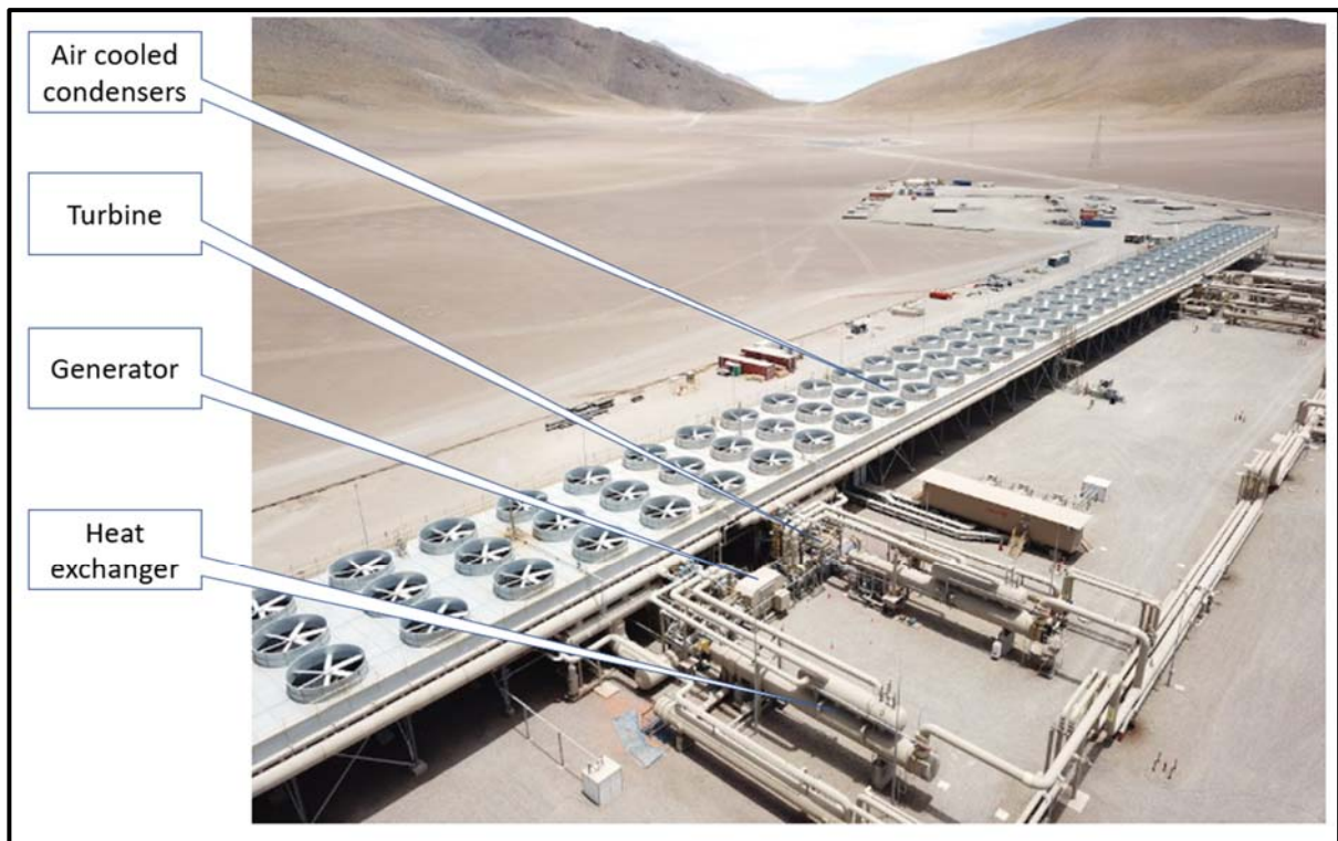
Figure 4.2: 48 MW Binary power plant, Cerro Pabellón, Chile. This plant is in the Atacama Desert in the Antofagasta region at an altitude of 4,500 masl (source: ThinkGeoEnergy).
