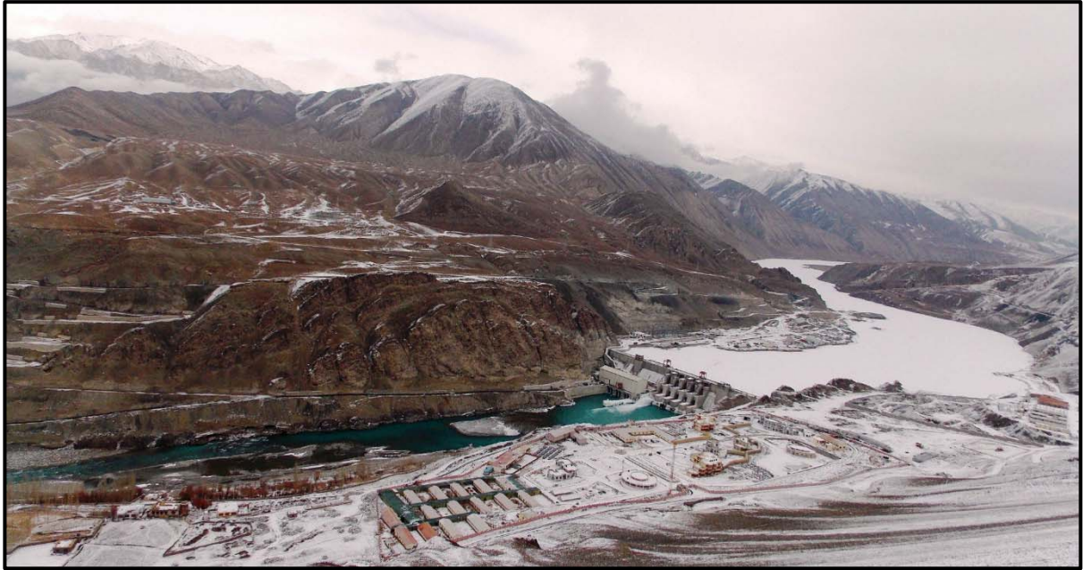
Figure 2.6: Aerial view of Nimoo-Bazgo 45 MW Hydro Project commissioned in 2013 (Wikimedia commons, 2013)
