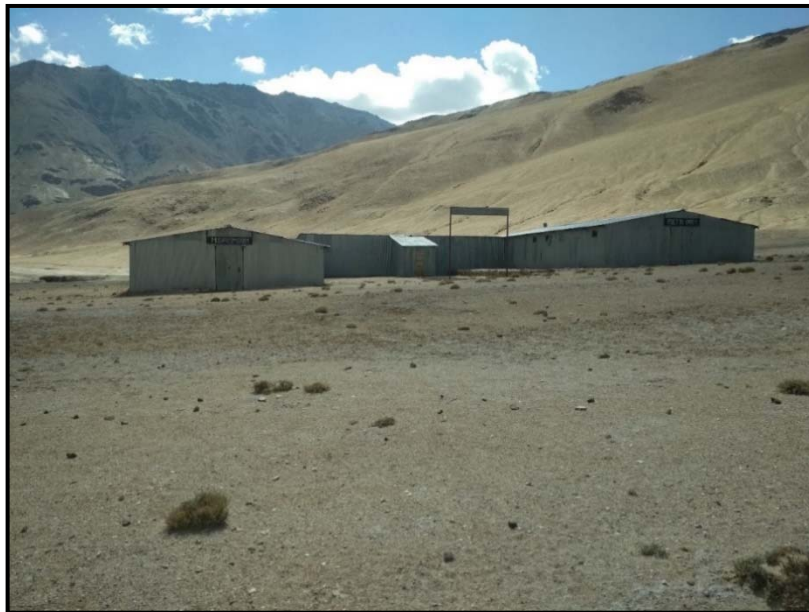
Figure 1.9: Present state of the demonstration poultry and mushroom farm at Puga which was successfully implemented by the Geological Survey of India in the 1970s but now abandoned.
