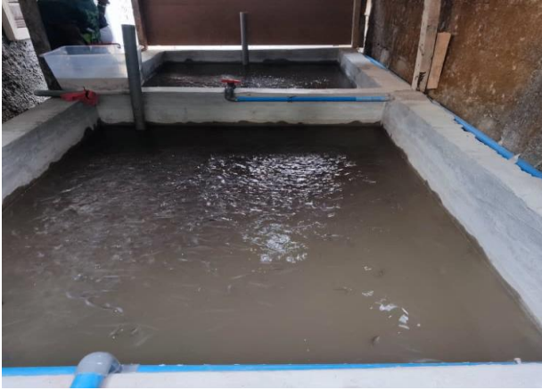
Newly constructed hatchery
