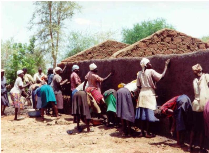
**Fig. 4.** Plastering of mud walls using decoctions from the husk of *Parkia biglobosa* (Photo: Margaret Shao 2002).
