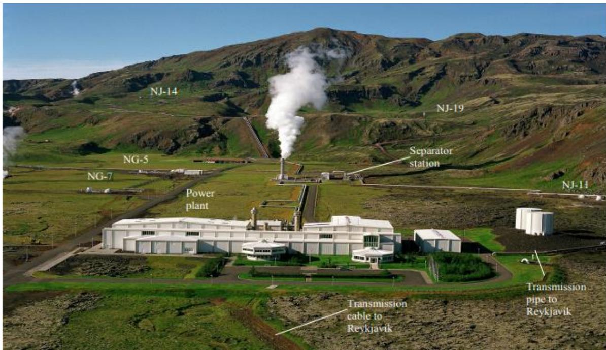
**Figure 12.** Overview of Nesjavellir geothermal plant site (Photo taken from Ballzus et al., 2000)
